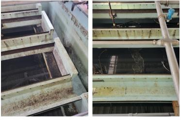
performance. During filter maintenance, crews remove algae, break down residual filter aids, break mud balls, and physically remove surface media contaminated with mud balls. The result is a clean filter that is ready for long efficient filter runs. With all the filters clean, crews can optimize treatment and get the most out of the filter runs.
